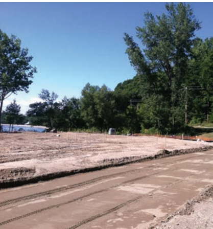
The Foundation's new pause place south of North Beach taking shape.
