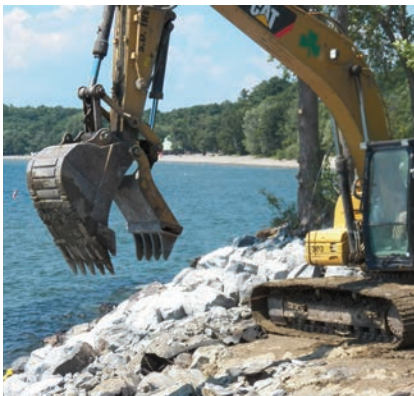
Shoreline stabilization near new Bike Path route.
